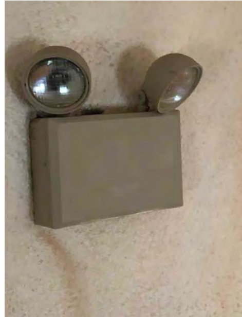
Dual Head Battery Pack Emergency Light in Great Hall; Textured Finish at Upper Wall (and Ceiling) is Sprayed Acoustical Finish from 2000 Renovation
