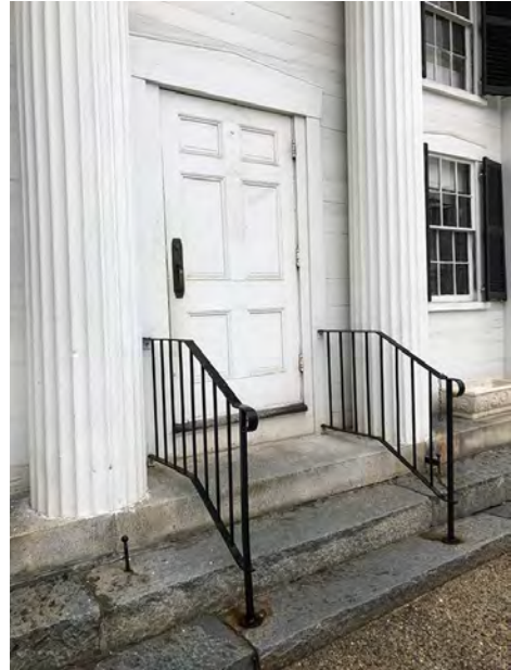
1848 Granite Steps to Entrance Stoop with Pair of Railings; Each Riser Varies in Height to Granite Plinth and to Final Step at Wooden Door Threshold to Foyer
