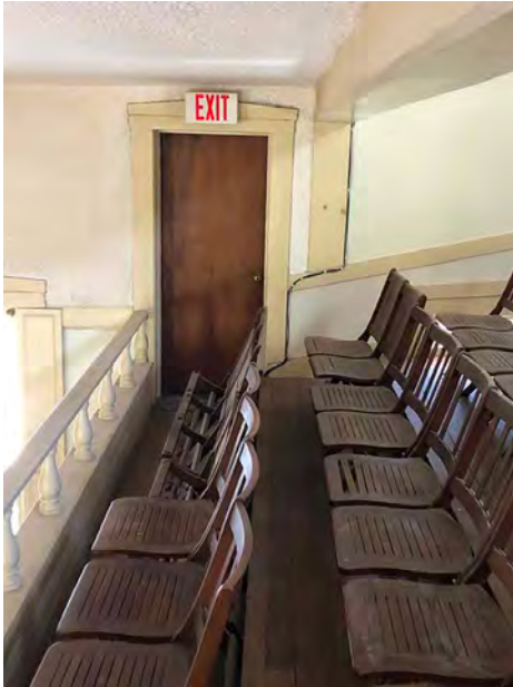
Front Rows of Balcony with South Exit to Fire Escape; Exit Door Operates with Extreme Difficulty; Second Exit Required if 50 or More Occupants in Balcony
