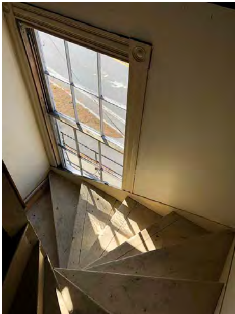
Looking Down 1895 Ell Attic Winder Stairs; No Handrails; South Wall Window at Great Road
