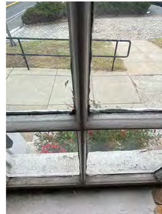
Original Window Sash with Typical Greek Revival Style Muntins
