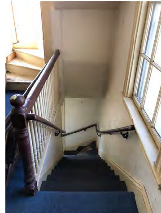
View in 1895 Ell from First Floor Down Stairs to Ground Floor with Winders at Turn Below
