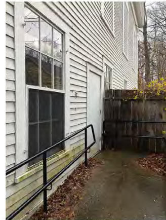
Existing "Accessible" Ramp at East Side of Building; Insufficient Landing and Door Clearances
