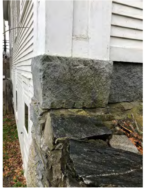
Tooling Marks in Granite at Base of NE Cornerstone; Retaining Wall in Foreground Toward Crescent Street
