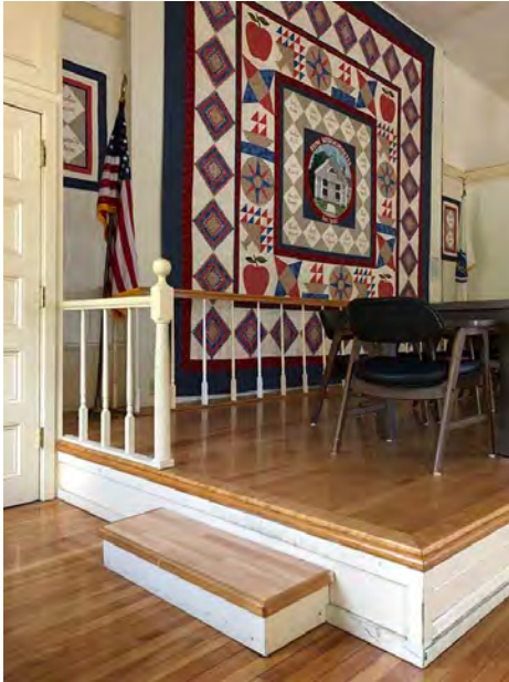
One Tread and Two Risers to Great Hall Stage at Each End of Stage; Stage not Wheelchair Accessible
