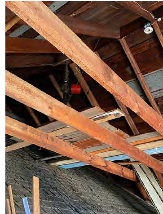
Exposed Collar Ties and Rafters of 1895 Ell in Attic
