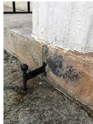
Iron Boot Scraper to Right of Entrance; Horizontal Scraper Portion Intact; Column Resting on Granite Plinth
