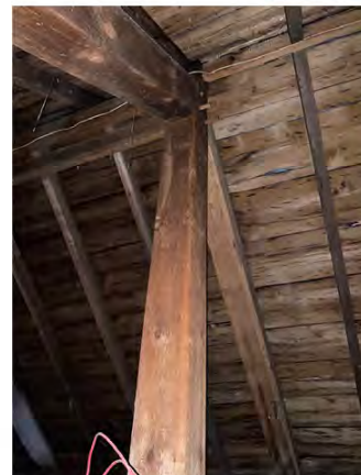
Timber King Post in 1848 Concealed Upper Attic Area
