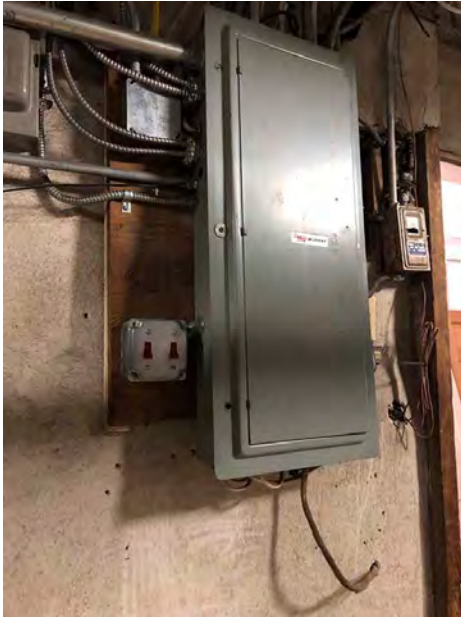
Electrical Service Panel at East Wall of Mechanical Room in Cellar
