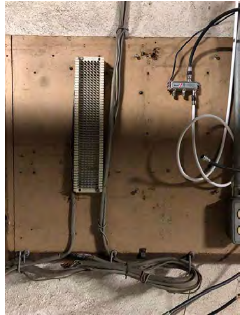
Patch Panel for Telephone and Cable Service at East Wall of Mechanical Room in Cellar
