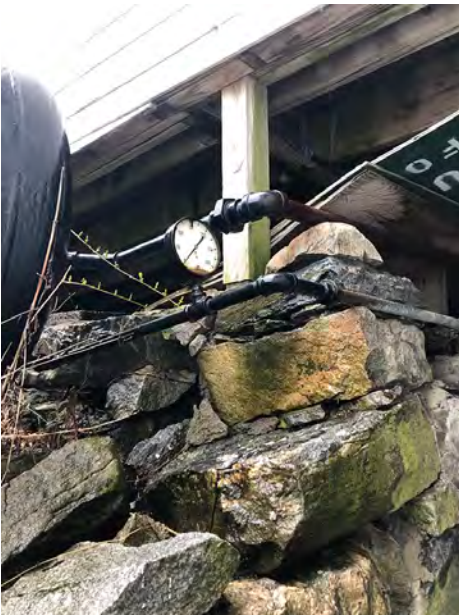
Wooden Post Bearing on Rubble Masonry at Ramp Structure to Side Entrance Adjacent to Abandoned Pneumatic Tank Serving Former Fire Alarm Notification System for Town
