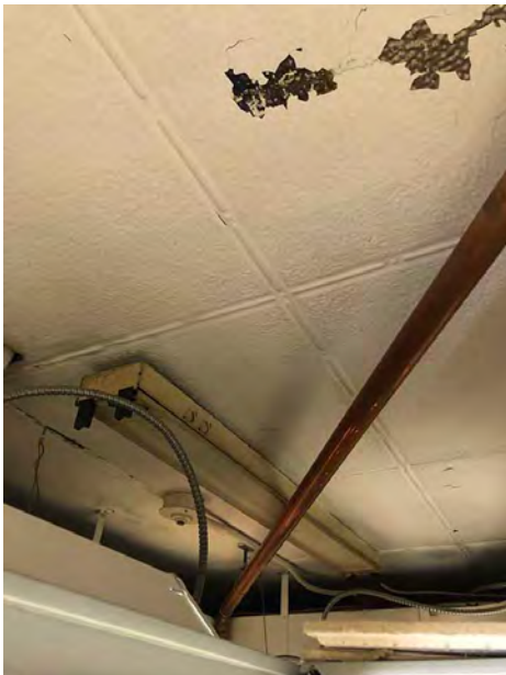
Copper Piping, Abandoned Light Fixture and Painted Tin Above Kitchen Acoustical Ceiling
