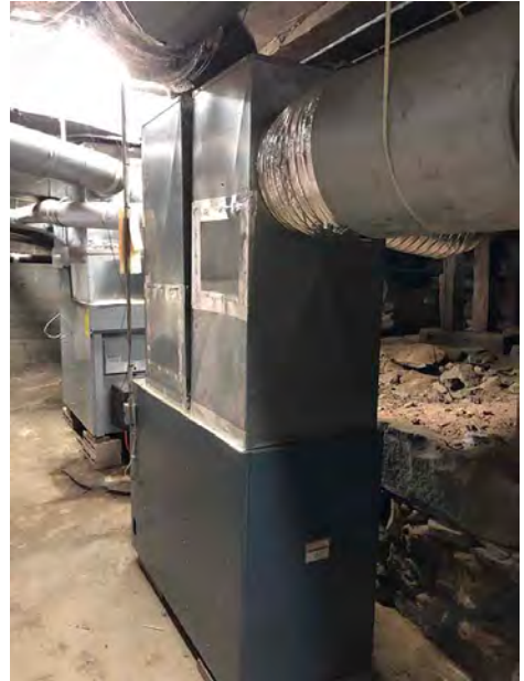
Pair of Oil-Fired Hot Air Furnaces in Cellar Mechanical Room; Existing Heating System
