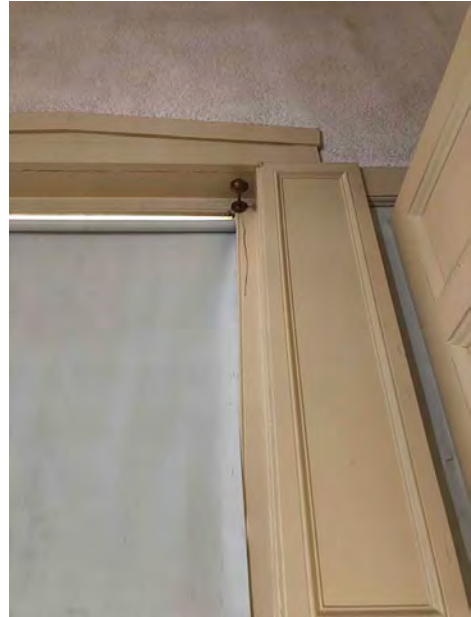
Great Hall Window Head Casing and Fixed Interior Shutters at Jamb; Former Drapery Hardware at Head
