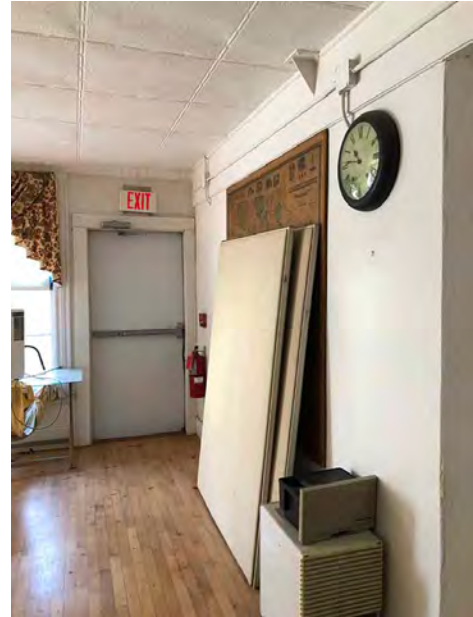
Exit Door to Exterior Ramp at SE Corner of Former Ground Floor Office Area; Strike Side Push Clearance at Door Inadequate on Interior Side of Exit; Pull Side Clearance at Exterior also Inadequate
