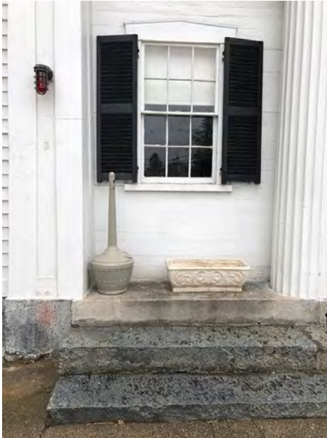
Flanking Window to Left of Central Entrance; Two Granite Steps up to Granite Plinth
