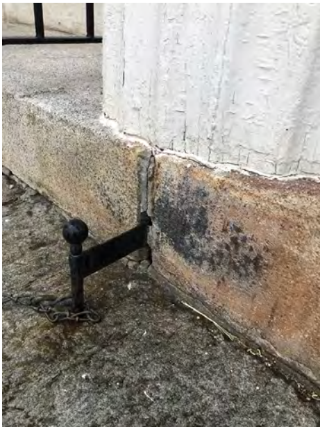
Intact Boot Scraper at South Side of 1848 Entrance; Base of Painted Fluted Column on Granite Plinth
