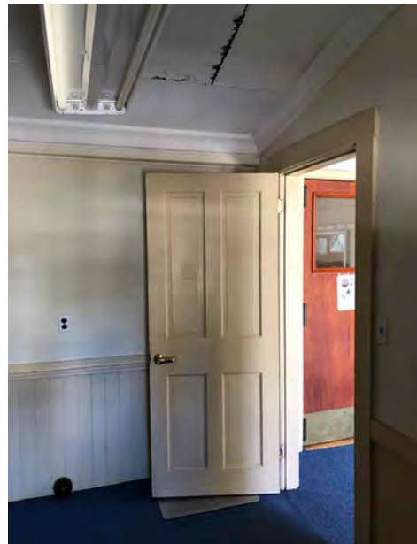
Four-Panel Door Leading from 1848 Entrance Foyer into Former Office at North Side of Foyer; 32" Wide Door not Handicap Accessible
