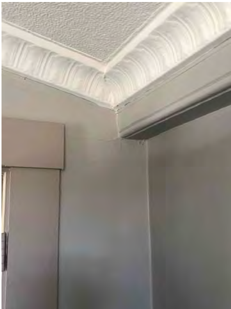
Detail of Painted Tin Crown Moulding at Ceiling of Former Office on South Side of 1848 Entrance Foyer
