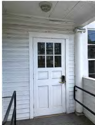
Existing "Accessible" Entrance to 1895 Ell with Insufficient Maneuvering Clearance on Pull Side; Project Proposes to Make Door Fully Accessible and Lower Threshold for Replacement of Ramp with Walkway
