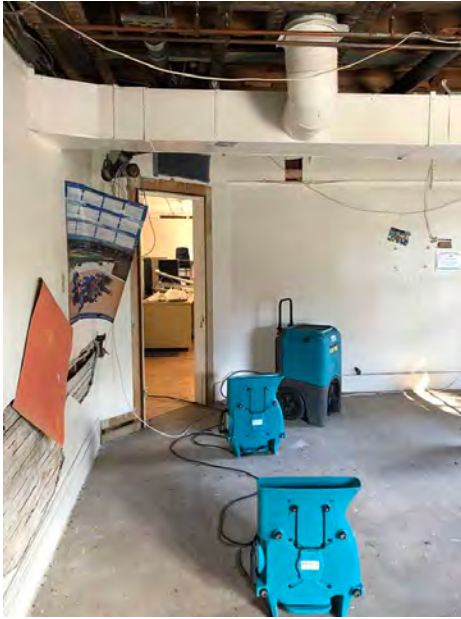
Painted Heating Ducts at Ceiling Serve Restrooms Above; Ceiling Removed Due to Recent Water Leak; Temporary Dehumidifiers (Blue) at Floor Level
