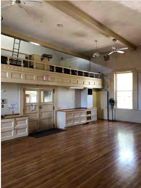
Great Hall and Balcony with Entrance Foyer Beyond; Built-in Cabinetry Added in 2000 Renovation; Duct Chases from Oil-Fired Furnaces Below; Attic Access Ladder Visible at Upper Left
