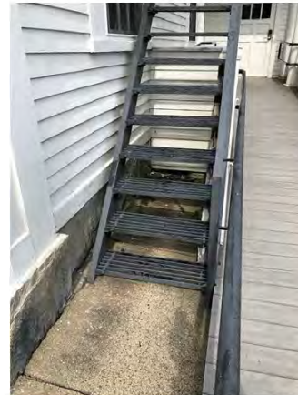
Lower Run of Fire Escape Stairs Separated from Adjacent Ramp Leading to 1895 Entrance Beyond
