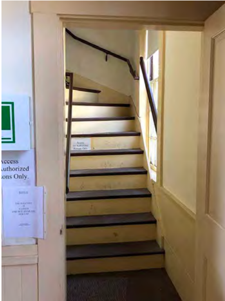
Stair Leading from Main Hall to Balcony in NW Corner; Discontinuous Handrails on Both Sides of Stairs
