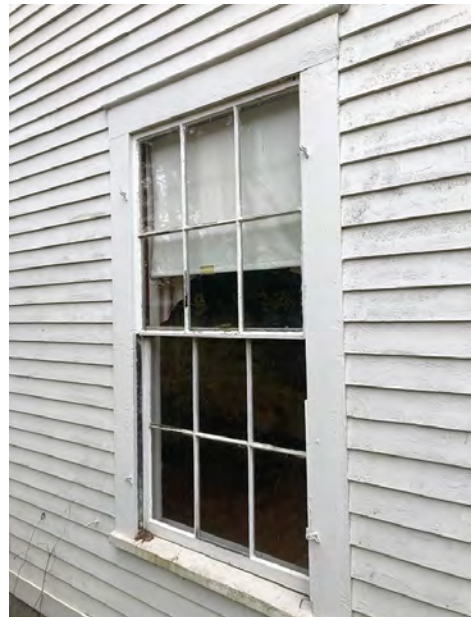
6-over-6 Wood Window Sash in East Facade of Ground Floor at 1895 Ell Addition; Painted Wood Clapboards
