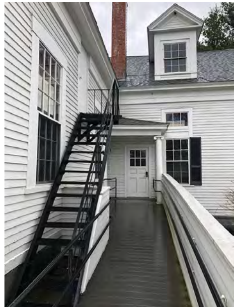
Accessible Ramp Heading East to Ell Entrance; Fire Escape Serving Balcony of Great Hall at Left; Dormer in 1895 Attic; Chimney Flue for Furnaces
