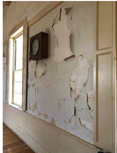
Peeling Paint at Plaster of Great Hall; Painted Wainscoting Below Windows and Acoustical Finish Above Windows; Wall-Mounted Clock on North Wall of Great Hall; Exterior Walls are not Insulated
