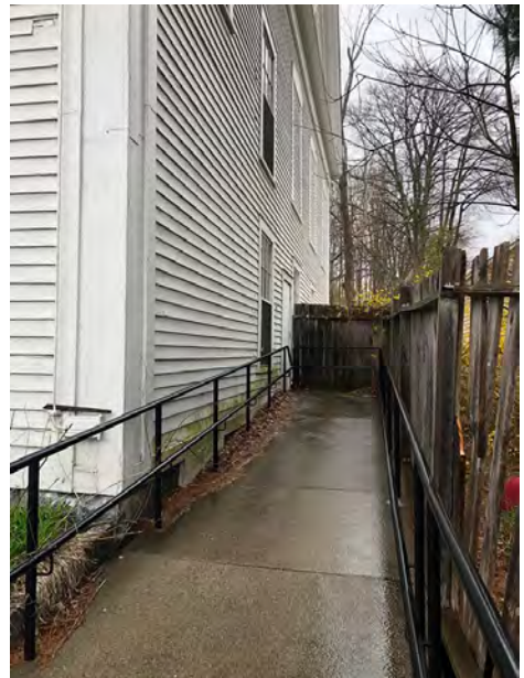
Accessible Ramp at East Side of 1895 Ell to Ground Floor Enters at Former Office Area; Ramp is on Abutter's Property with Permission; Upper Landing Area & Door Clearances Inadequate
