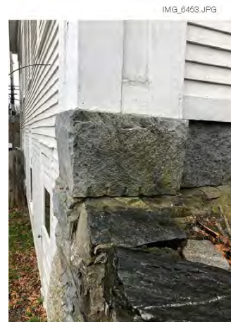
Detail of Granite at Northeast Cornerstone Showing Tooling Marks from Quarry
