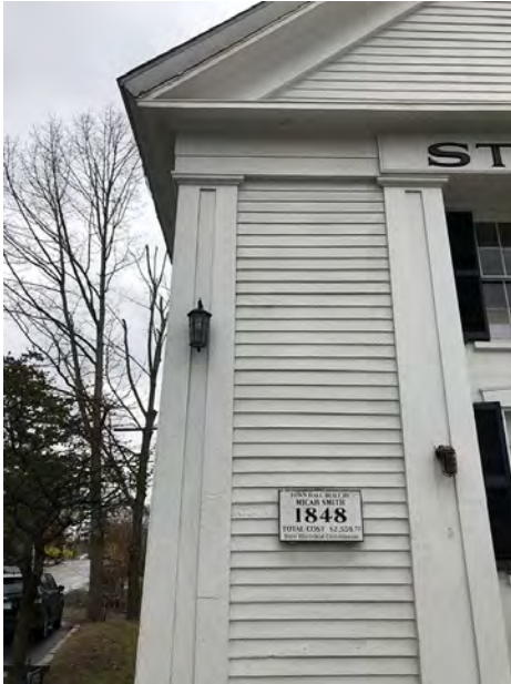
Pilasters & Clapboards at NW Corner of Primary Facade
