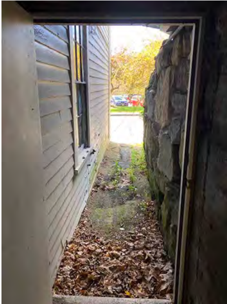
Looking South Thru Service Alley Toward Great Road from Cellar Door; Bulging Stone Retaining Wall at Right; Blocked Kitchen Window at Left
