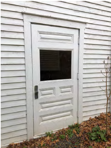
Inoperable Door from Ground Floor in East Facade Blocked by Elevated Height of Finished Grade
