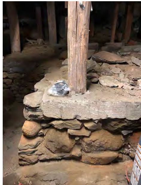
Timber Post on Concrete Pad over Rubble Masonry
