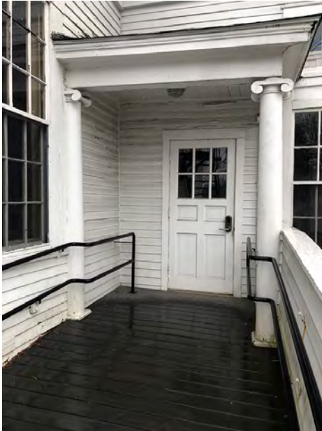
1895 Ell Entrance to Stair Hall at Accessible Ramp; Inadequate Strike Side Clearance at Pull (18" Required); Chimney at Interior Restricts Clearance on Hinge Side
