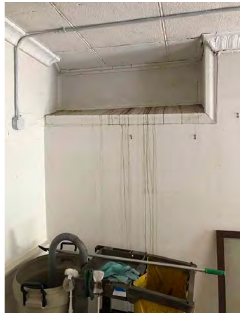
Evidence of Water Infiltration at Blocked Cellar Sash in NW Corner of Former Ground Floor Office; Plaster Finishes Conceal Rubble Stone Foundation Wall at North Side
