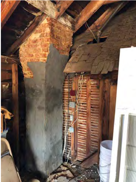
Parged Brick Furnace Chimney in NW Corner of 1895 Attic Adjacent to Former Exterior Wall of 1848 Town Hall; Original Clapboards of South Wall Removed
