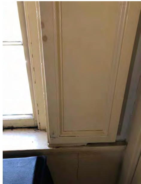
Interior Shutter Fixed in Place at Great Hall Window Appears to be Solely Decorative - Not Wide Enough to Cover Half of the Window
