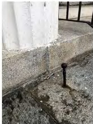
Iron Boot Scraper to Left of Entrance; Missing Horizontal Scraper Portion; Column Resting on Granite Plinth
