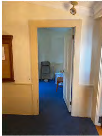
Typical Flat Interior Casings in 1848 Foyer; Rush Wood Wainscoting; Painted Tin Ceiling
