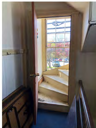
Attic Stairs in Ell Originating at First Floor; Winders at Each of Two Turns in Stair Run
