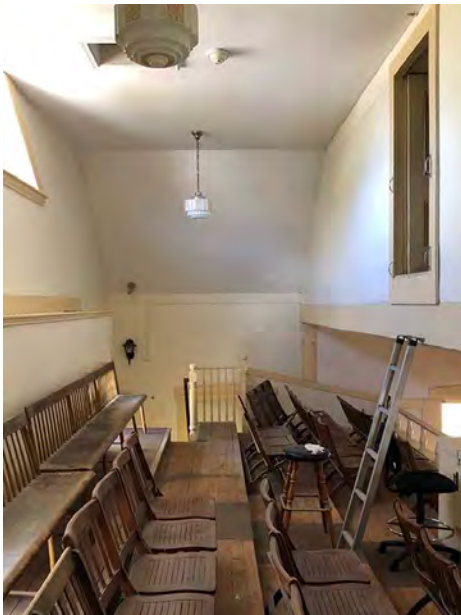
Looking North in Balcony Area Toward Stair; Attic Access Thru Hatch in Wall at Right via Aluminum Ladder Hitched in Place & Removable
