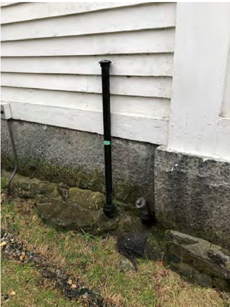
Fuel Oil Fill & Vent at North Facade Adjacent to NW Corner
