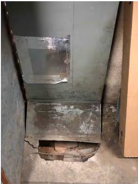
Combustion Air Opening in Cellar Slab at Base of Duct Along East Wall Adjacent to Furnaces
