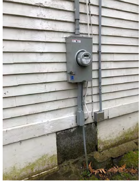
Electrical Meter at North Facade Near NW Corner; Existing Service is 100-Amp, Single-Phase, 120/240-Volt
