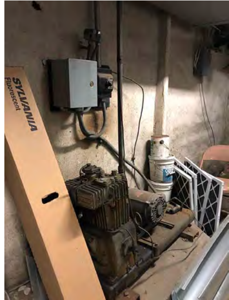
Abandoned Compressor in Mechanical Room for Former Air Horn Fire Alarm Notification System
