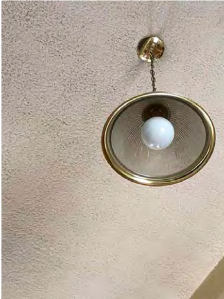
Textured Ceiling Finish Reduced Reverberation in Great Hall; Acoustical Finish and Light Fixtures Referenced in "Stow-Info" Historical Society Newsletter of February 2000
