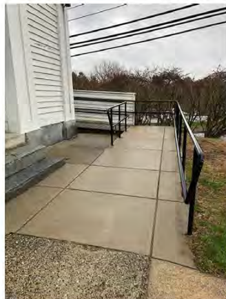
Existing Confusing Duality of Accessible Ramp at Right Adjacent to Fire Escape Exit Route at Left
