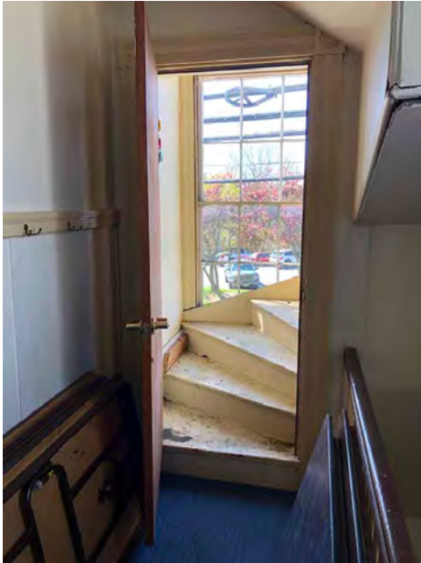
Winder Stairs from First Floor of 1895 Ell to Attic; No Handrails at Stair
