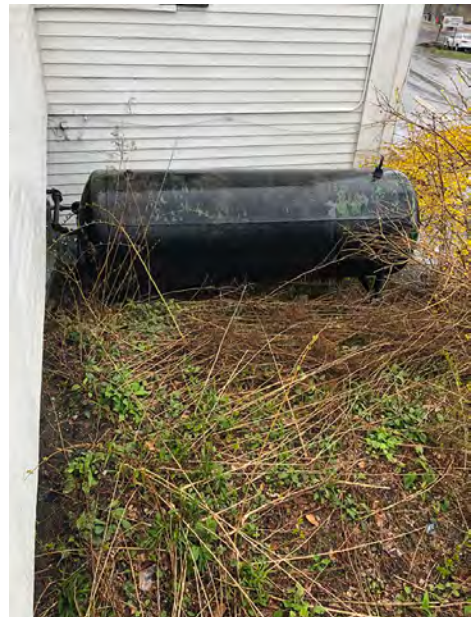
Pneumatic Tank in South Yard for Former Fire Horn; Abandoned Horn Penetrated Roof for Town Notifications
