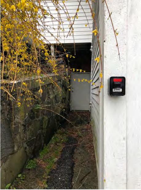
Service Alley to Cellar Entrance Adjacent to 1895 Addition; Bulging Rubble Stone Retaining Wall at Left Side of Alley; Knox Box for Fire Department Keys at SW Corner of Ell
