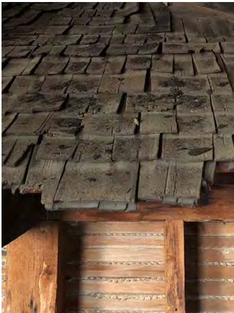
Detail of Wood Shingles at 1848 Roof Surface; Wood Lath and Plaster Keys in Great Hall Wall Where Plaster was Replaced in 1895 when Ell was Added
