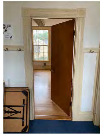
Typical Belly Band Interior Casings with Rosettes in 1895 Ell at Windows at Doors; No Wainscoting and Painted Plaster Ceilings; Maple Flooring Below Carpet
