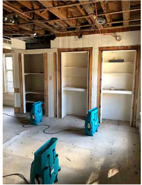
Dehumidifiers in Former Office Below Restrooms Following Recently Repaired Water Leak; Former Ceiling Removed to Expose Wood Framing
