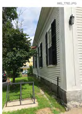
North Facade of Building Facing Crescent Street; Continuous Granite Plinth Typical of Greek Revival
