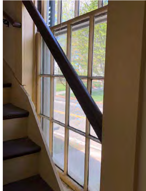
Guard Rail Adjacent to Balcony Stair at Window Opening
