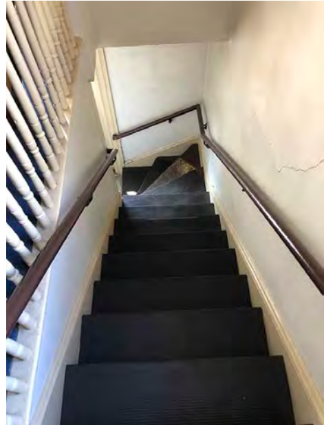
Looking Down Winder Stairs in 1895 Ell from First Floor to Ground Floor Level
