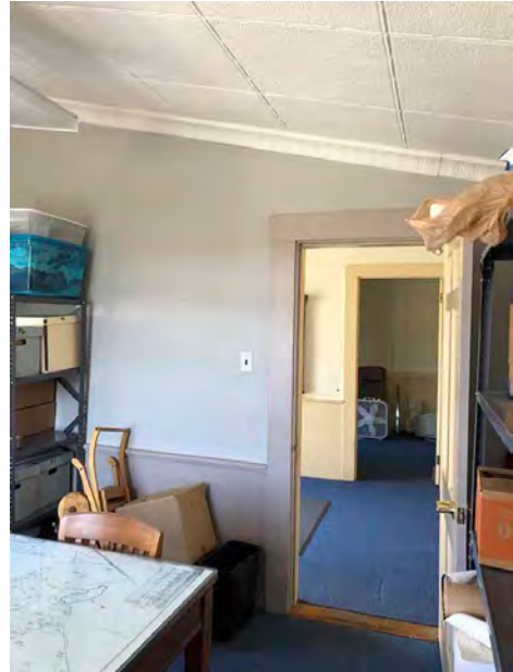
Looking North in Former Office Adjacent to 1848 Entrance Foyer Beyond; Sloping Tin Ceiling of Balcony Above; 32" Wide Door not Handicap Accessible
