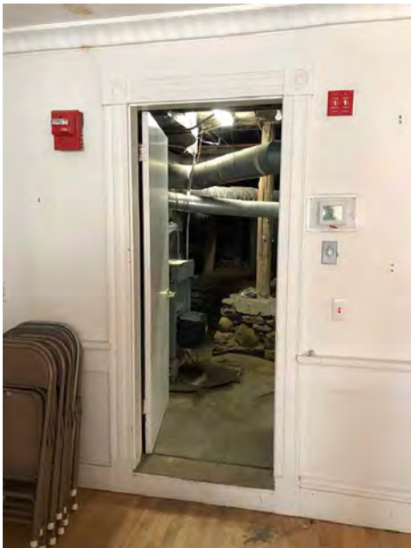
Raised Threshold at Door from Ground Floor Former Office Area to Mechanical Room in Cellar
