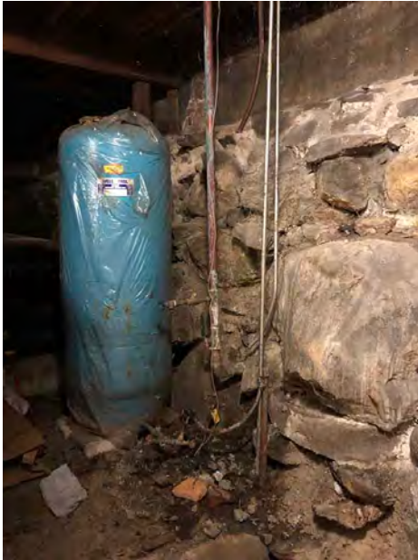
Pressurized Well Tank Adjacent to Electrically Grounded Water Service at North Rubble Foundation Wall
