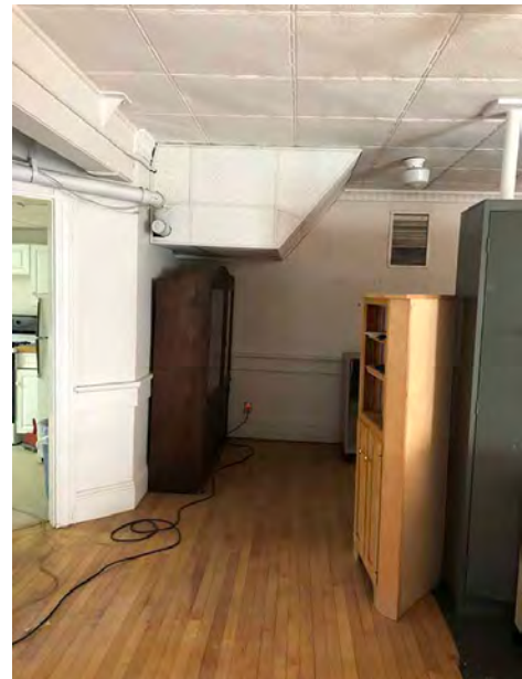
SW Corner of Former Office Area Adjacent to Kitchen; Acoustical Tile Ceiling Soffit Conceals Oil-Fired Furnace Flues to Brick Chimney at Left
