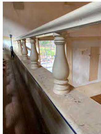
Original Spandrel and Balustrade at Open Side of Balcony
