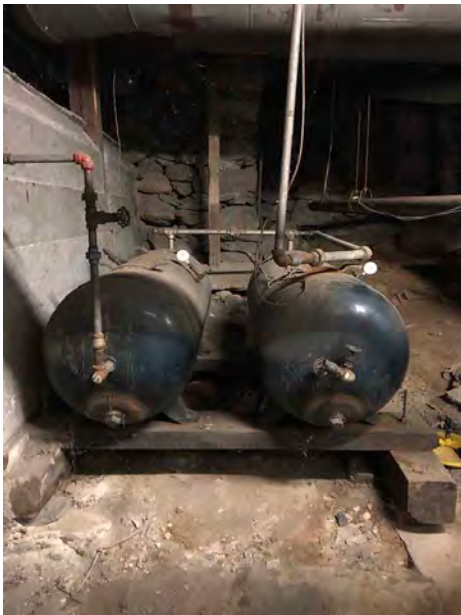
Abandoned Interior Air Tanks for Former Fire Horn System Adjacent to South Foundation Wall; Concrete Buttress Added to South Stone Wall
