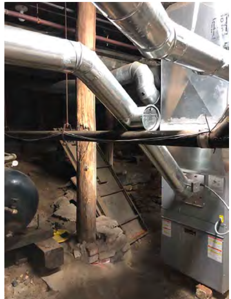
Hewn Timber Log Post Adjacent to Oil-Fired Hot Air Furnace
