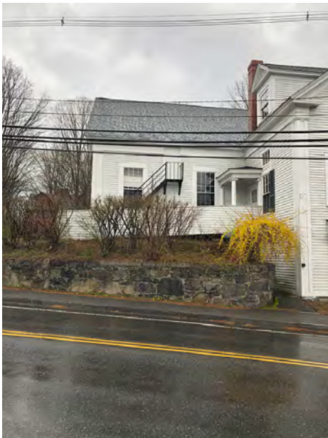
South Facade of 1848 Portion with 1895 Addition at Right; Low Clapboard Wall is Guardrail for Accessible Ramp; Fire Escape Stair Exit from Great Hall Balcony
