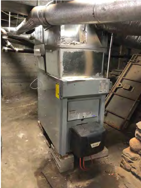
One of Two Oil-Fired Hot-Air Furnaces in Cellar
