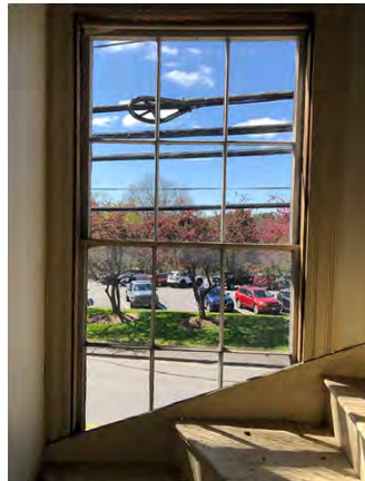
Attic Stair Adjacent to Window in South Facade of 1895 Ell with Original Sash to be Restored
