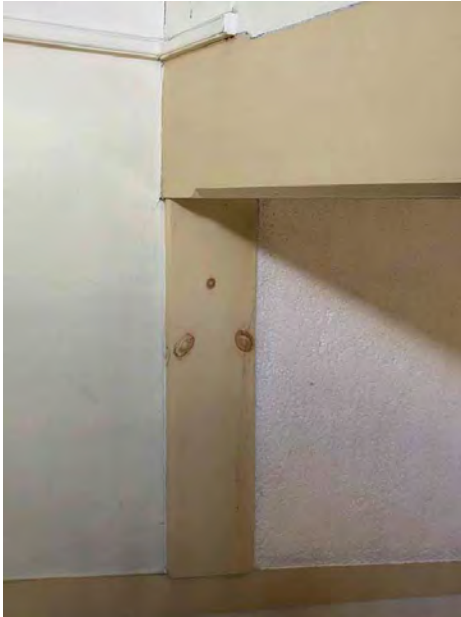
Painted Pilaster and Chamfered Beam at Intersection of Attic Framing to North Wall of Balcony at Main Hall; Low Headroom at Beam in Balcony (68" Above Tier 2); Pilaster Added as a Stop for Sprayed Acoustical Finish
