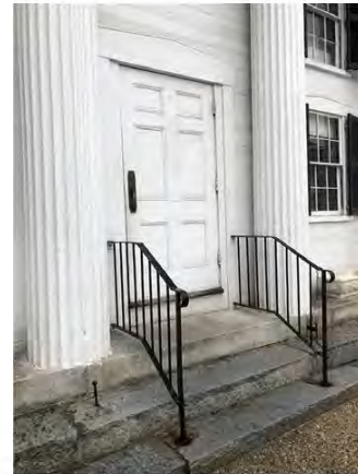
Front Entrance with Two Granite Steps up to Plinth, Followed by Step up at Wood Threshold to Floor Level; Ruted Columns Rest on Granite Plinth 9" Below Floor
