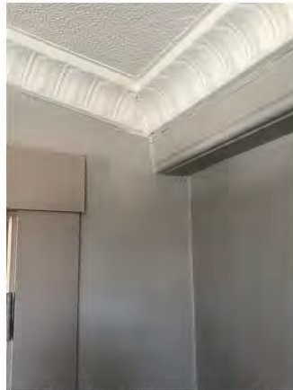
Detail of Painted Tin Ceiling and Crown at First Floor Office Below Balcony of Great Hall Above
