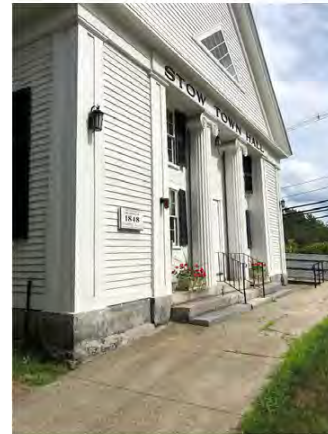
Historic Front Entrance on Granite Plinth; Project Proposes to Re-set Lower Two Steps to Re-establish Consistent Riser Heights to Plinth
