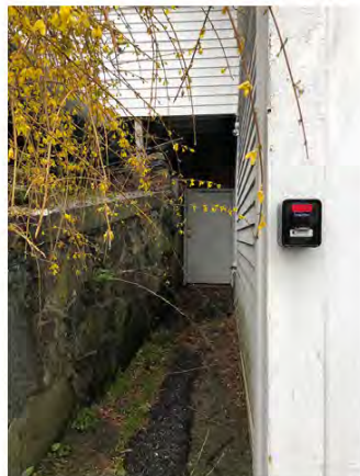
36" Wide Service Alley Between Stone Retaining Wall and Adjacent 1895 Ell; Entrance to First Floor Above; Walkway to be Widened for Accessible Entrance to Ell
