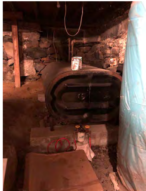
Active Fuel Oil Tank Adjacent to North Foundation Wall Serves Pair of Hot-Air Furnaces for Heating System
