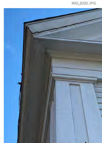
Detail of Corner Pilaster, Frieze, Rake & Clapboards Typical of Greek Revival Style
