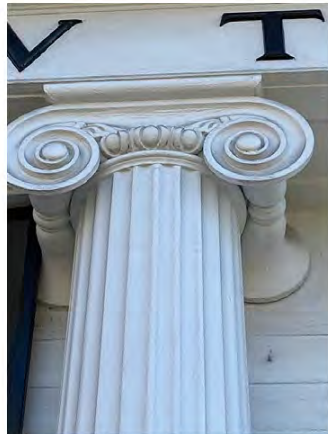
One of Two Fluted Wooden Column with Ionic Capitals at Front Facade; Pair Frames Entry & Supports Pediment
