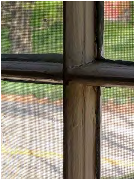
Greek Revival Muntin Profiles in Great Hall Window Sash; Half Screens Visible at Exterior of Lower Sash
