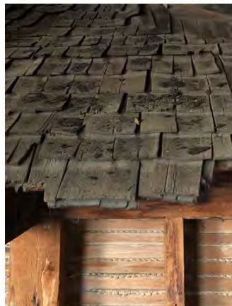
Exposed Former Wood Shingles on South Slope of Original Roof Visible in 1895 Attic of Ell
