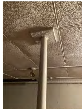
Textured Painted Tin Ceiling in Office Area of Ground Floor; Simple Clad Column Capital Typical Where in Finished Area
