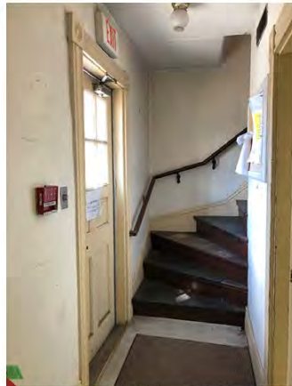
Winder Stairs in 1895 Ell at Ground Floor with Adjacent Exit Door Leading to Great Road
