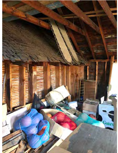
Siding Removed Revealing Lath & Plaster of 1848 Wall; Wood Shingles Remaining at South Slope of 1848 Roof
