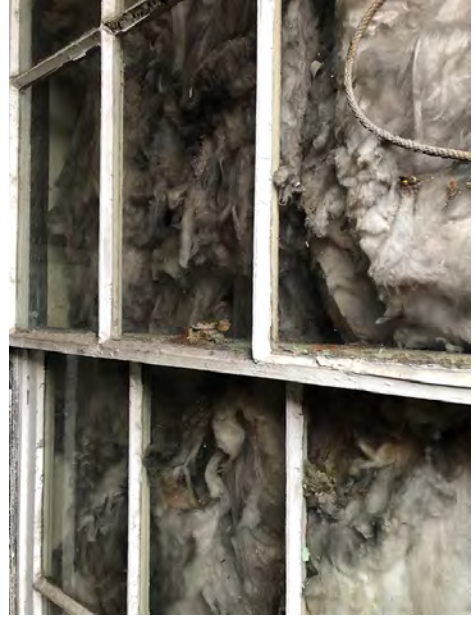
Insulation in Blocked Window Opening of Kitchen in West Wall of 1895 Ell Adjacent to Service Entrance; Window Not Visible from Interior of Kitchen
