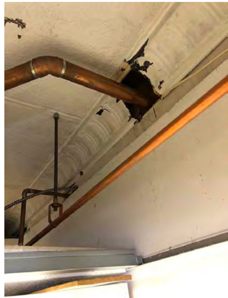
Copper Piping Penetrating Tin Crown Above Kitchen Ceiling
