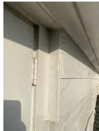
Original Dual Board Frieze Interrupted by Fire Escape Exit Door Opening will be Restored
