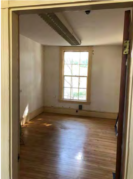
Former Office at First Floor of 1895 Ell Adjacent to Stair Hall; Window in East Wall; Louvered Strip Fluorescent Light Fixture; 32" Wide Door not Handicap Accessible
