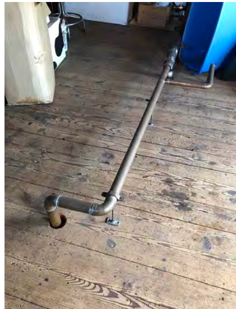
Plumbing Vent from Restrooms at First Floor and Kitchen at Ground Floor Installed Exposed Above Floor Level of 1895 Ell Attic
