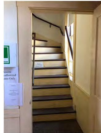
Stair from Great Hall to Balcony; Winders at Turn and Discontinuous Railings; Proposed Project to Replace Railings for Continuity
