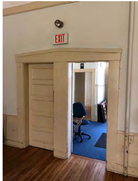
Pair of Doors at Exit from Great Hall to 1895 Ell; Head Casing Detail Matches Windows of Town Hall; Doors 32" Wide not Handicap Accessible
