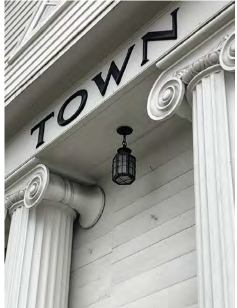
Ionic Volute Capitals on Fluted Columns of Pediment; Sign Band on Added Wood Board Across Pediment
