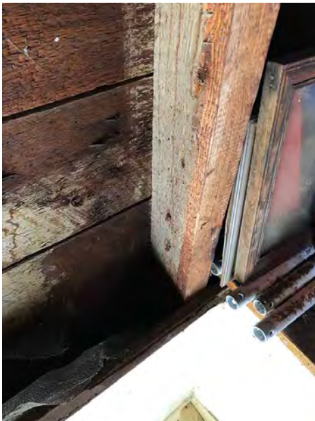
Exposed Wood Stud and Board Sheathing at NW Corner of 1895 Ell Attic Stair; Plaster Finish Stops at Attic Floor Level
