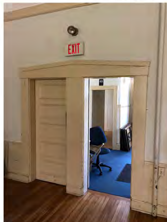
Pair of 32" Doors from Great Hall into 1895 Ell; Project to Retain Original Framed Opening and will Provide Accessible Door in Center with Equal Sidelights
