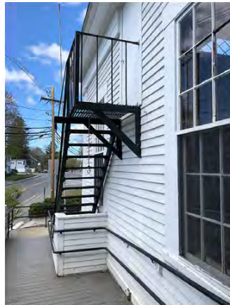
Exterior View of Fire Escape Serving the Balcony
