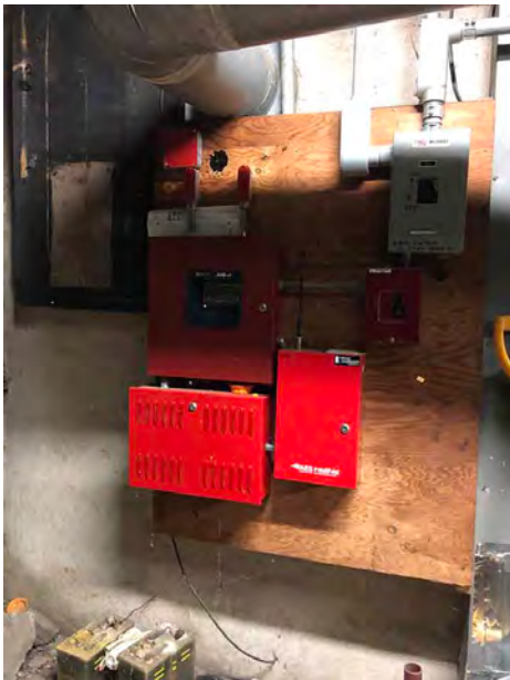
Fire Alarm Control Panel Components in East Wall of Mechanical Room
