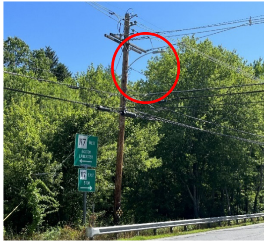
Figure 6: Single light at the intersection of Great Road at Hudson Road.
