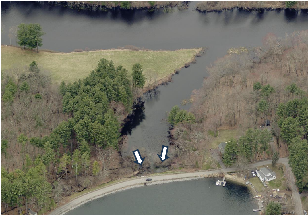
Figure 6: West facing view of Lake Boon Dam, Bailey's Brook, and confluence with Assabet River (EagleView, 2019). The remnant downstream embankment sections separated by the narrow breachway are indicated by arrows.
