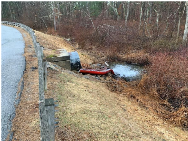
Figure 5: Photograph (March 2021) of dam embankment downstream slope and discharging spillway.
