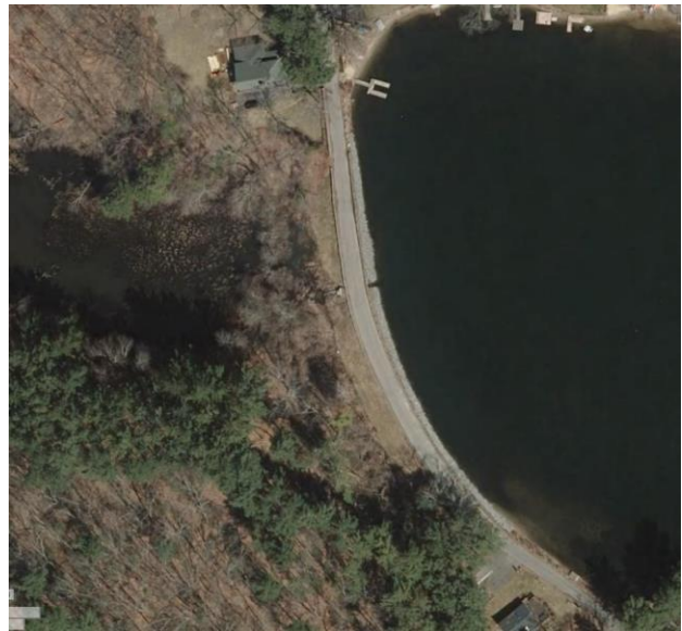
Figure 4: Aerial photograph of Lake Boon Dam (MassGIS, 2019 Imagery).
