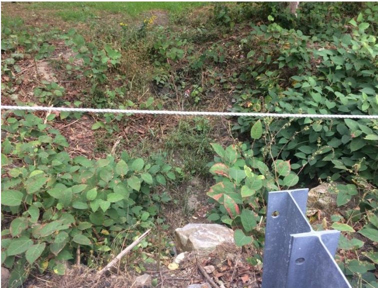
Fig. 4 Dry culvert crossing at 2 Marlboro Road
