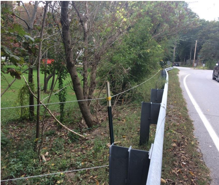
Fig. 3 Frontage at 2 Marlboro Road
