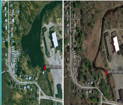
Whittenton Mill Dam was removed in 2013
