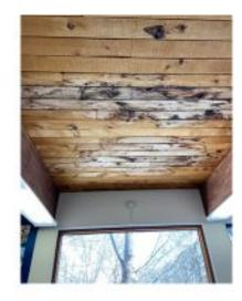
Recurring roof leak damage on the second floor of the 1970's addition
