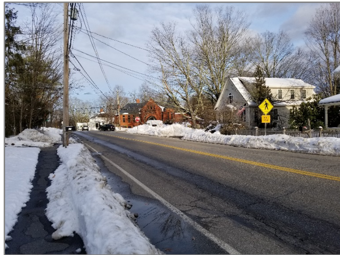
A portion of Crescent Street that includes sidewalks in fair condition
