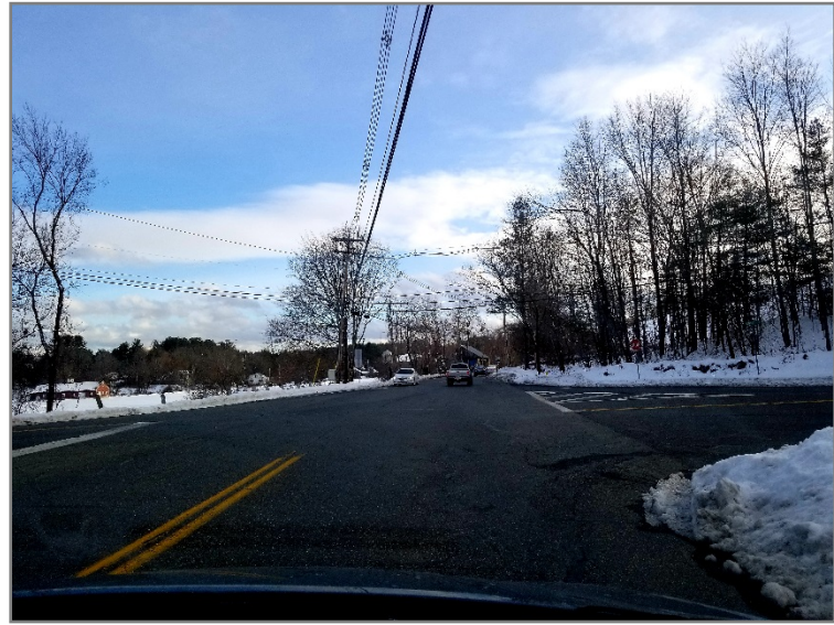
Wide travel lanes and intersection that lack bicycle facilities and shoulders at the intersection of South Acton Road, West Acton Road, and Boxboro Road.
