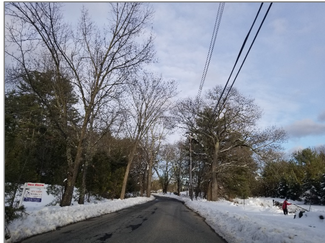
A portion of Old Bolton Road that will include sidewalk construction on the NB side.
