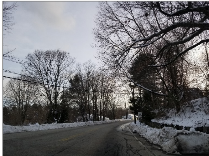
A portion of Crescent Street that is included in the sidewalk construction proposal.
