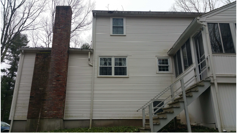
EXISTING CONDITIONS - PHOTO
