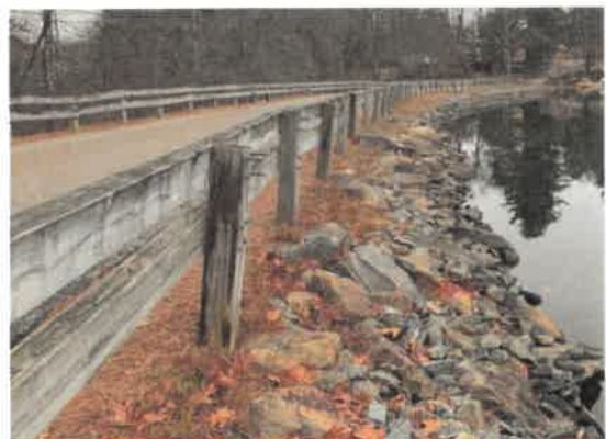
Figure 1: Existing timber guardrails along Barton Road.
