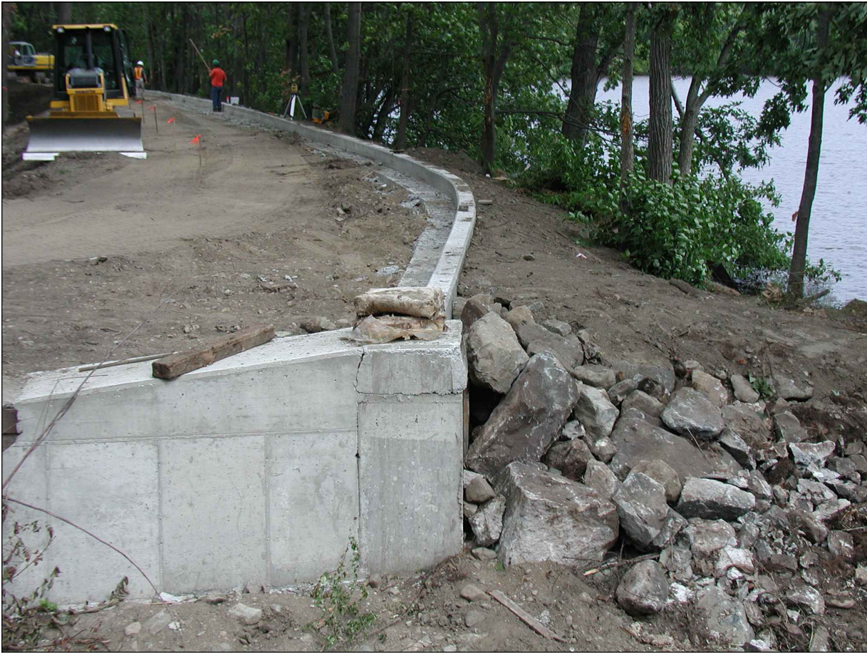
CONCRETE BEAM CAP CONSTRUCTED OVER SHEET PILE WALL (ARLINGTON RESERVOIR DAM, 2005)
