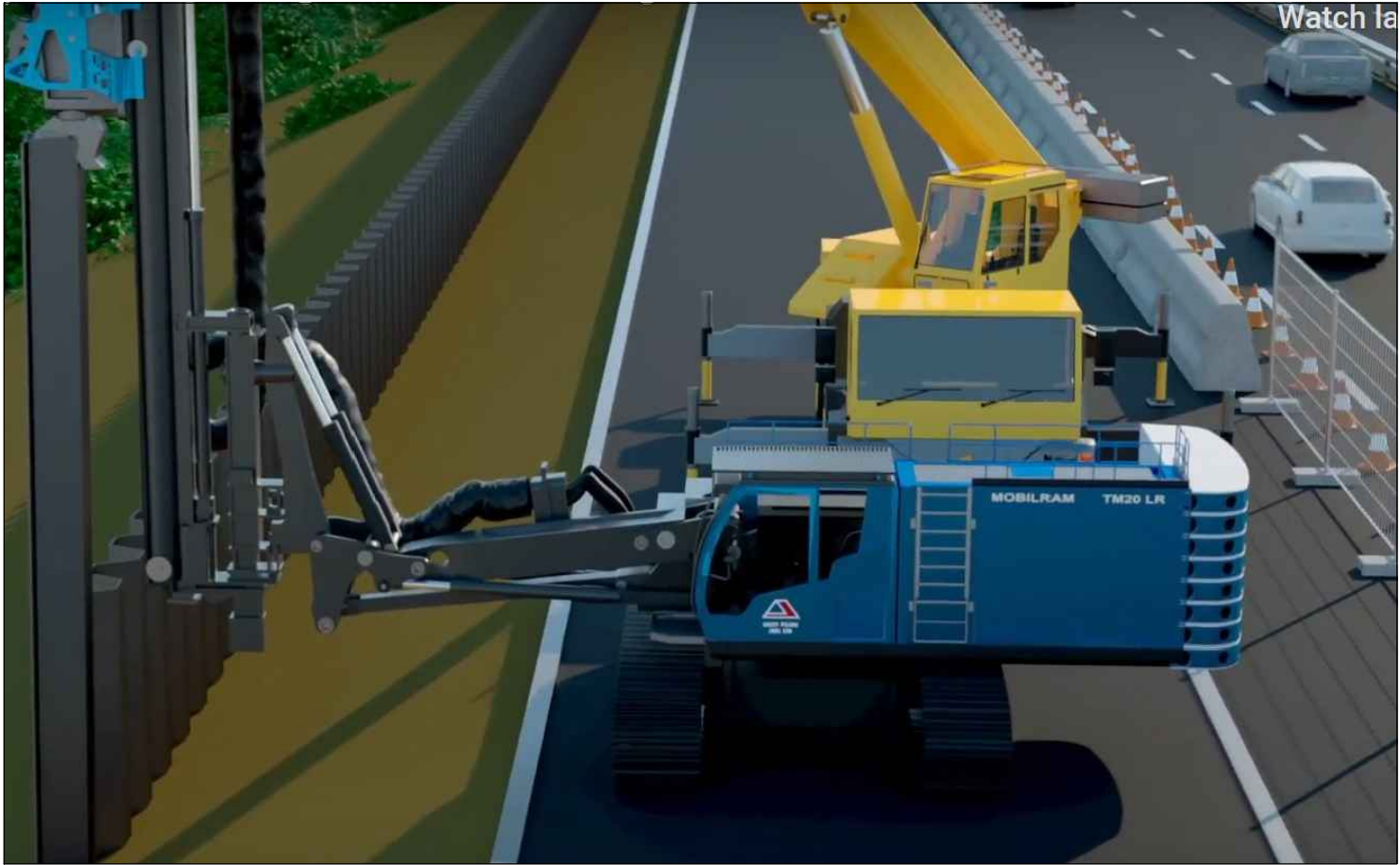
ILLUSTRATION OF CLEARANCE REQUIRED FOR FIXED-MAST PILING INSTALLATION EQUIPMENT
