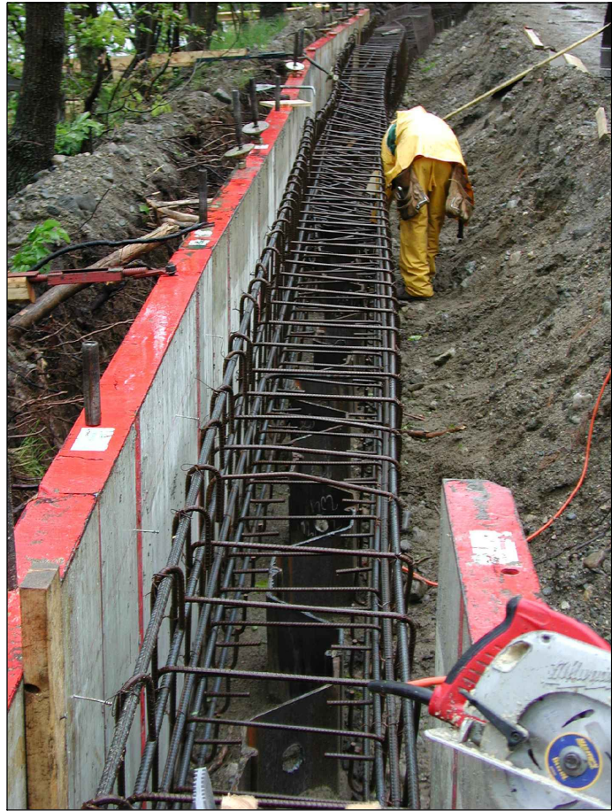
CONCRETE BEAM CAP UNDER CONSTRUCTION (ARLINGTON RESERVOIR DAM, 2005)
