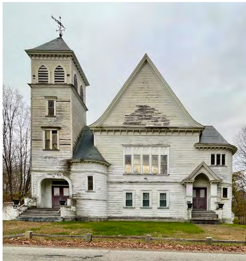
An historic church building in Gleasondale Photo Credit: JM Goldson
