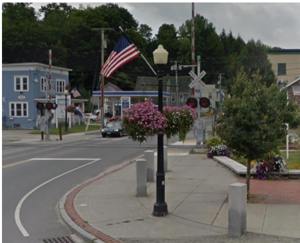
PEDESTRIAN SCALE LIGHTING AND STREET TREES, RANDOLPH, VT
