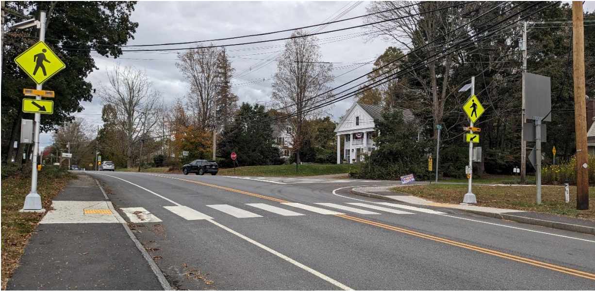
High visibility crossing by Town Hall at Crescent Street, with Rectangular Rapid Flashing Beacons (RRFBs) and new accessible ramps.
