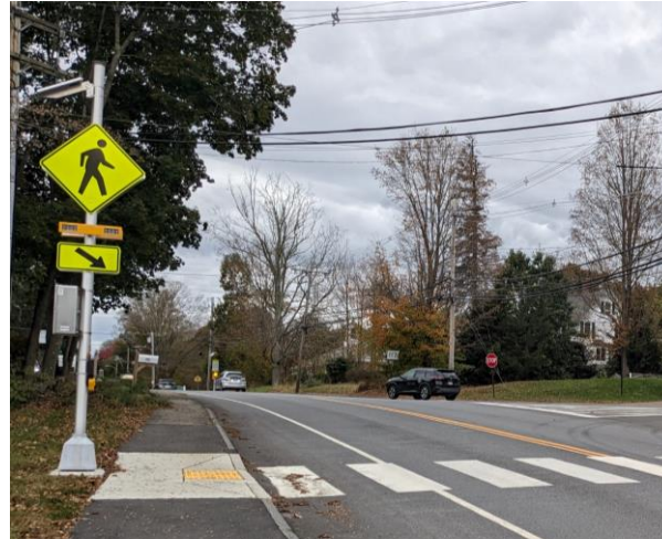
RECTANGULAR RAPID FLASHING BEACON, STOW, MA
