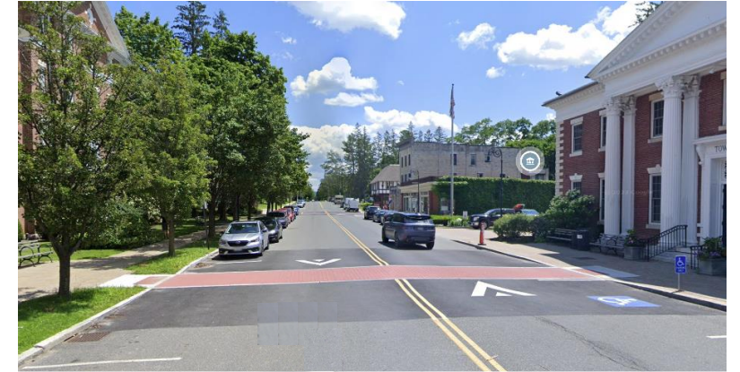
RAISED CROSSWALK, LENOX, MA
