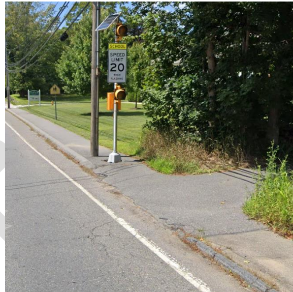
Narrow sidewalk on Great Road is interrupted by a utility pole and signage. Source: Google Maps.
