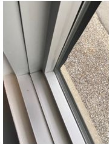
ALUM FRAME WITH INSULATING GLAZING
