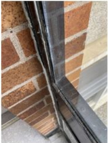
STEEL FRAME WITH SINGLE GLAZING
