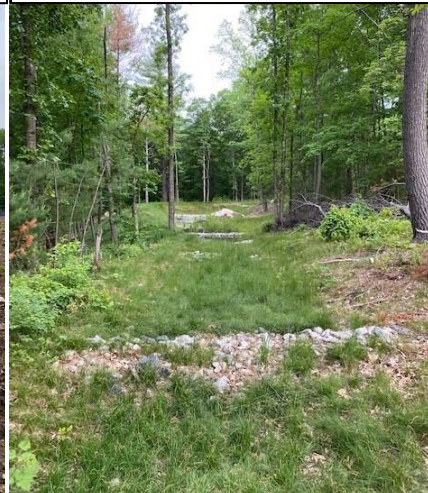
(G) Grassed swale routing stormwater to Stormwater Management Area #1.
