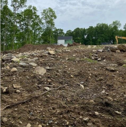
(E) Lot #2 has been cleared & grubbed for proposed house & septic area. No erosion or washout was observed downgradient of Lot #2
