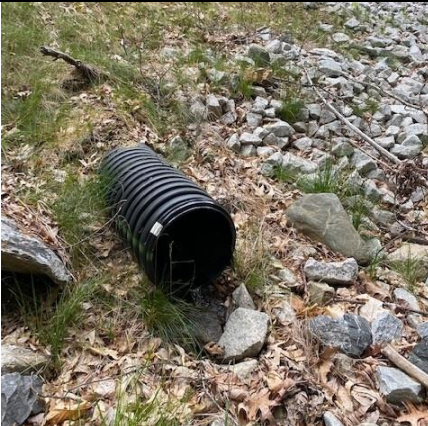
(U) Outlet Culvert for Stormwater Management Area #2. Flow was observed from Outlet Culvert #2, no erosion or scour was observed.
