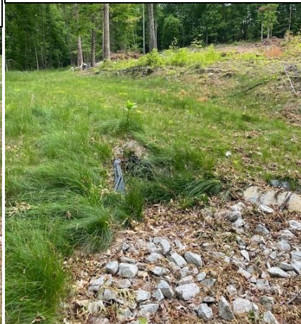
(O) Flared End section. Rip-rap was installed at culvert outfall to prevent erosion & scour.
