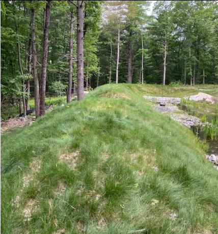
(M) Typical Check Dam in grassed swale.
