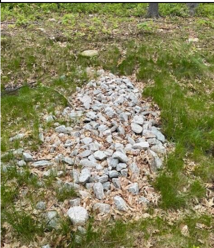
(M) Typical Check Dam in grassed swale.
