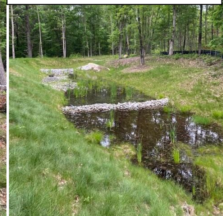
(H) Standing water observed in Stormwater Management Area #1. ~1.5" of rainfall occurred from 5/29-5/31.
