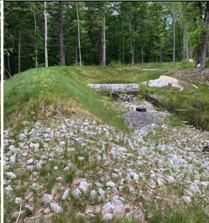
(N) Standing water was observed upgradient of rip rap check dam. Water was observed flowing toward Stormwater Management Area #1.
