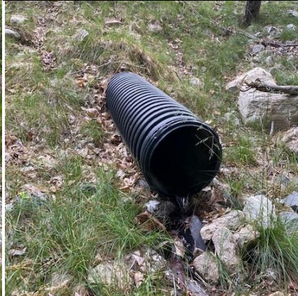
(O) Flared End section. Rip-rap was installed at culvert outfall to prevent erosion & scour.
