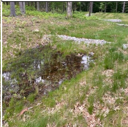
(N) Standing water was observed upgradient of rip rap check dam. Water was observed flowing toward Stormwater Management Area #1.
