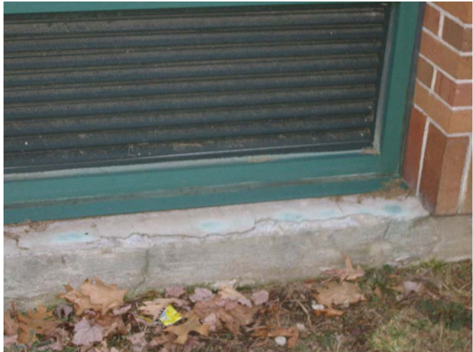
Concrete sill deterioration at existing curtain wall at grade.
