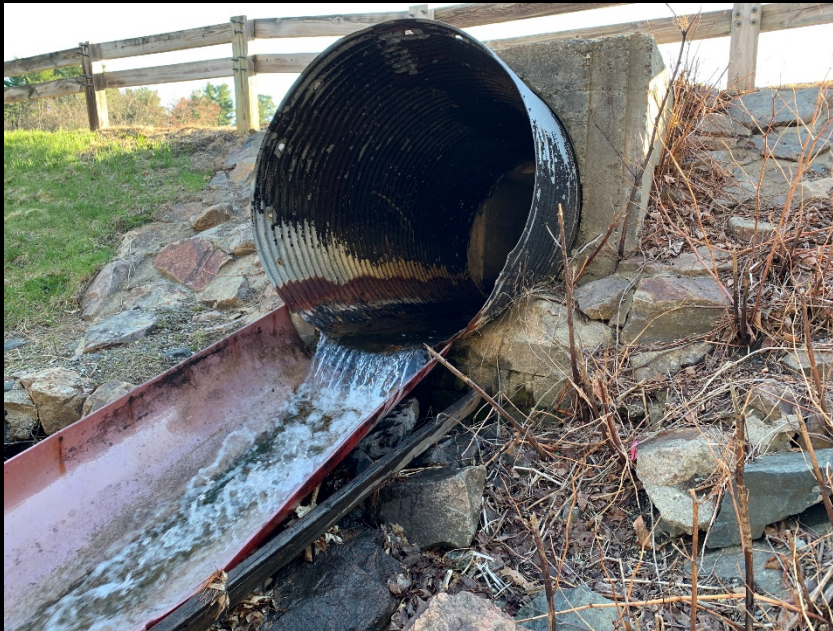
Spillway outlet structure in disrepair
