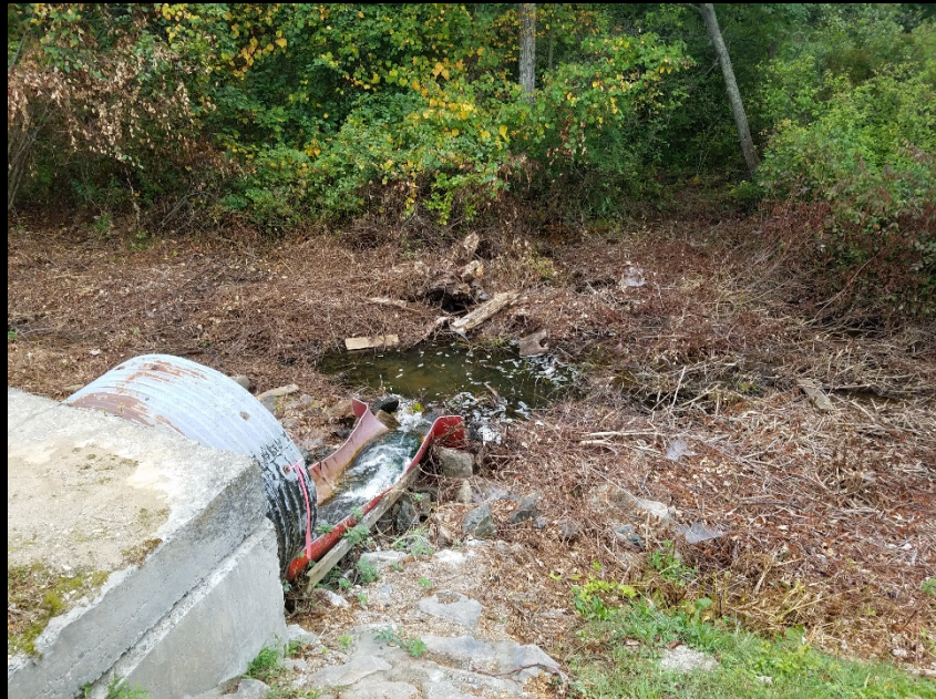
Scour hole below spillway along downstream toe
