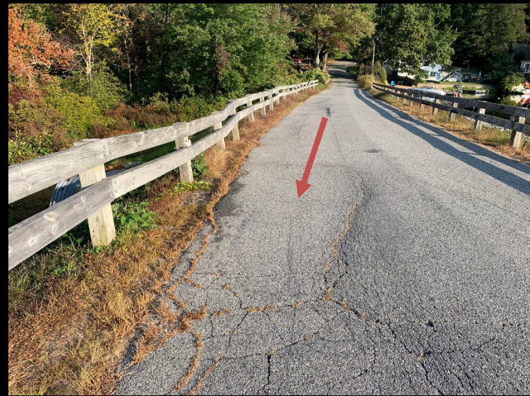
Evidence of embankment instability
