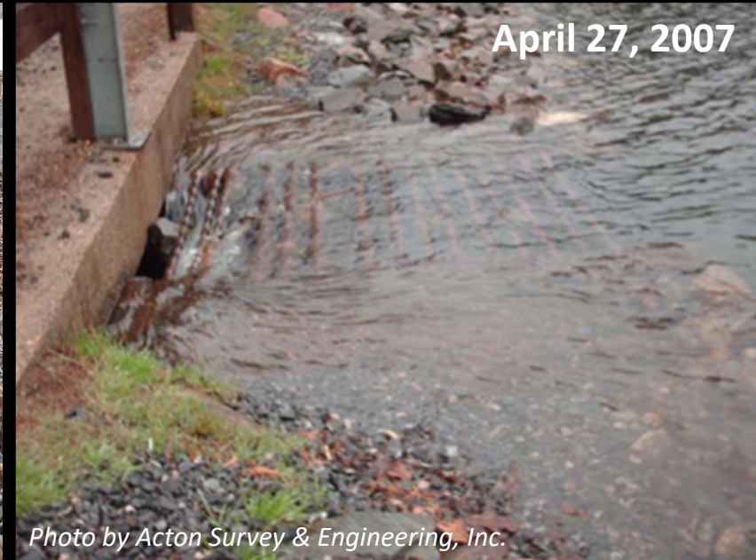
Inadequate spillway capacity / overtopping risk
