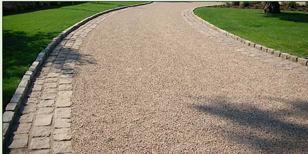
2 STYLES OF CHIPSEAL DRIVEWAYS ON PRIOR PROJECTS. CHIPSEAL IS NOT PERMEABLE. IT IS A THIN LAYER OF STONE CHIPS THAT ARE ROLLED WITH OIL ONTO AN ASPHALT BASE
